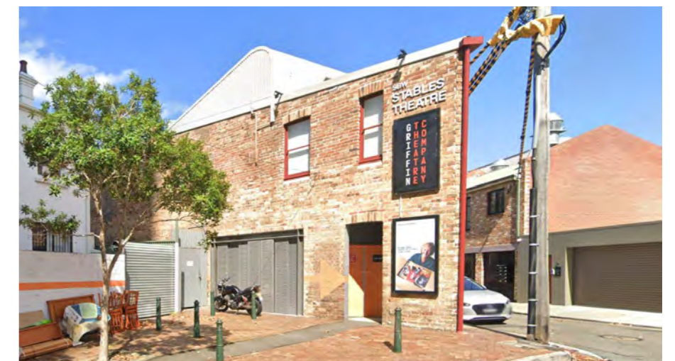
The footpath is widened to form a paved area to the east of the site. A right of way separates the building from its neighbours. This is accessed via a tall metal gate.
